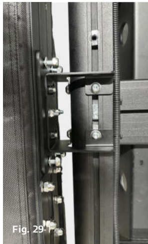
Tightening the nuts
